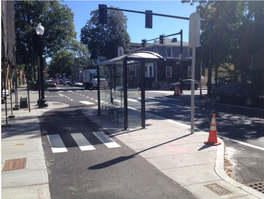
Bus Boarding Island
